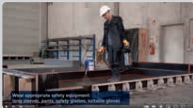
Application of concrete release agents
