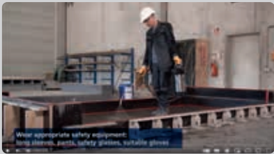
Application of concrete release agents
