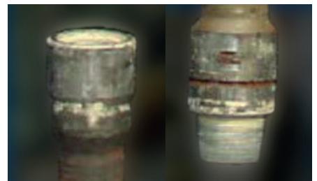
Figure 6 Connection after break-out
