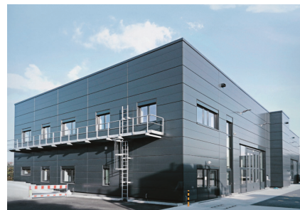
Test field in Mannheim
